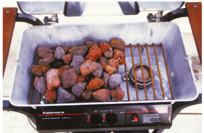
Above The burner installed in barbecue
