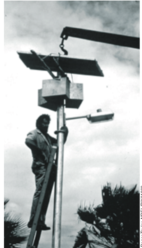
Worker installing a grid-independent, PV-powered street light.
