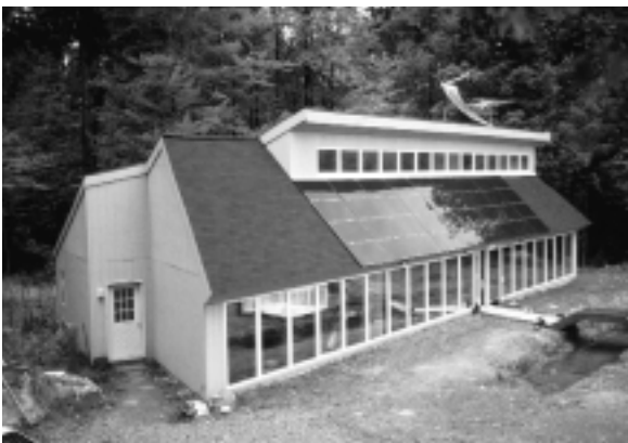
This home in Hopewell, New Jersey, demonstrates the effectiveness of off-grid photovoltaics, solar thermal water heating systems, and passive solar building design.
