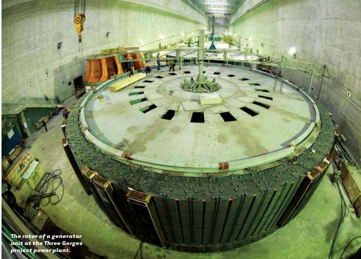
*The rotor of a generator unit at the Three Gorges project power plant.*
